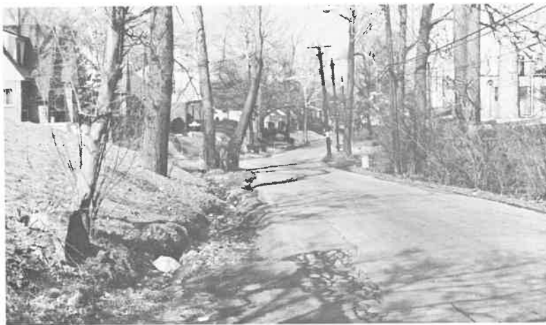
Street conditions in some arteries are deteriorated and the lack of curbs and sidewalks is creating pedestrian and vehicular problems.
