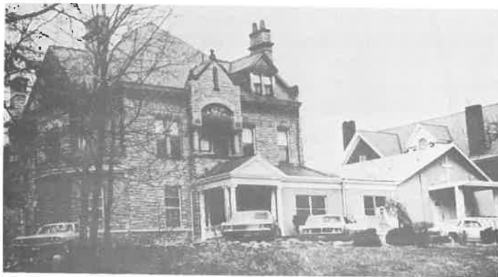
Conversion of a large old single family home to institution, disregarding aesthetic and environmental compatibility while destroying its original character.
